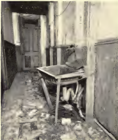
FIG. 100.—A hall and sink as the Department found them.
